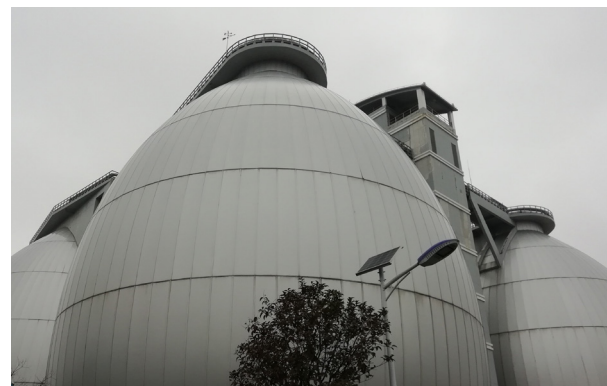
Digestion towers at a Chinese municipal wastewater treatment plant.
