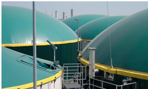
The Willingshausen biogas plant, with a plant capacity of 800 Nm<sup>3</sup>/h and an annual production of 9.1 million Nm<sup>3</sup> of biogas and 3.5 million Nm<sup>3</sup> of biomethane.
