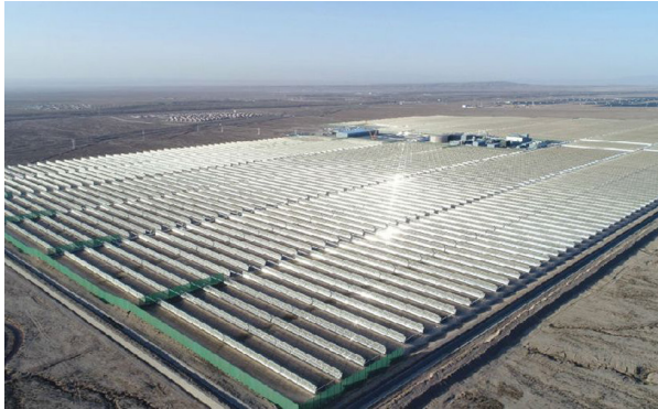
The first commercial CSP power plant in China: 50 MW CGN Delingha with 9h of storage and 9120 EuroTrough collectors.
