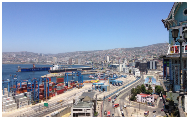
The complex infrastructure of a port (Valparaíso, Chile) can become a particular hazard if, for example, freight containers are swept away and driven inland by tidal waves.
