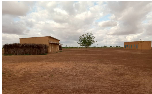
School building for the construction of pilot systems.
