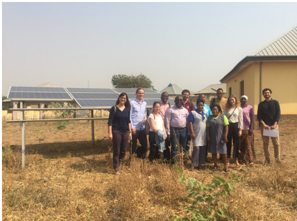
Solar system Dakwa PHC.
