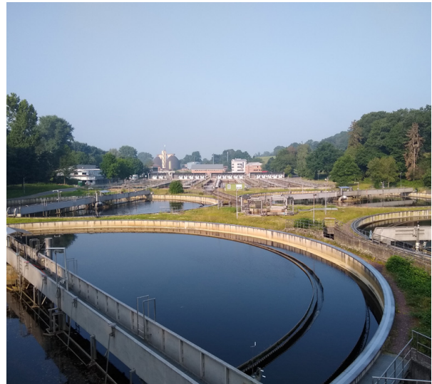
Aachen-Soers waste water treatment plant.
