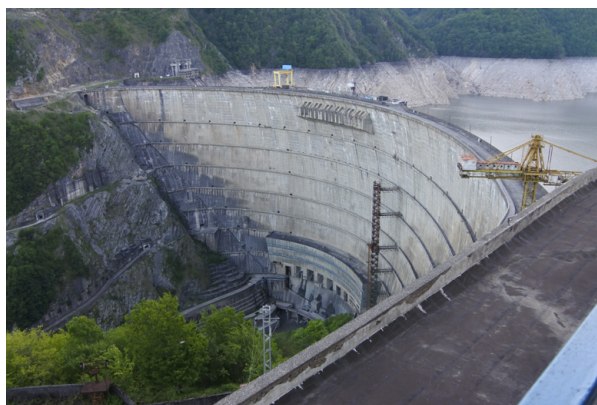
The 277 meter high arch dam of the Enguri Dam in Georgia.
