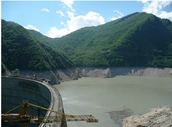
Compared to other dams, Enguri Lake has a very high annual water level fluctuation of approx. 100 meter.
