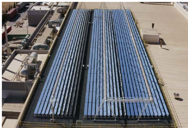
Solar thermal energy for the generation of industrial process steam.
