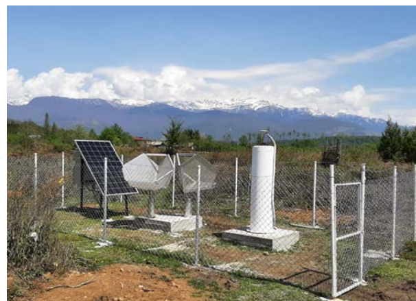
Geodetic station for the acquisition of data from the fields of seismology, geodesy, photogrammetry and water management, geomechanics.
