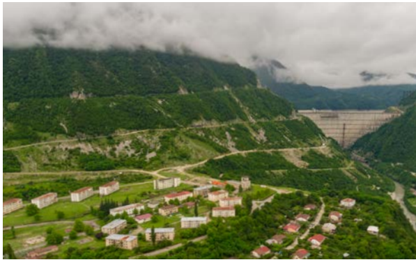
The 277 meter high arch dam of the Enguri Dam in Georgia.
